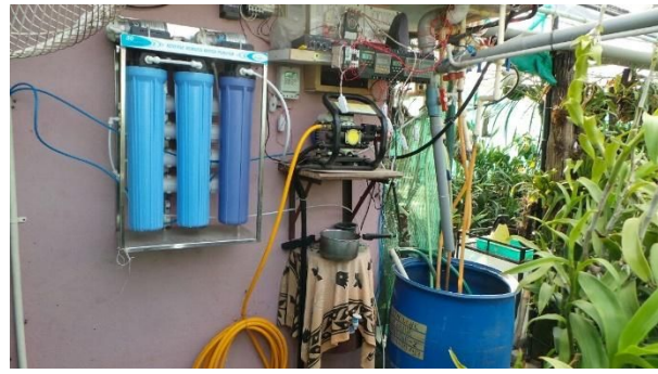
RO water system, softening of water & automation.
